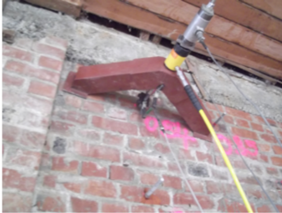
Figure 1: The steel frame testing set-up including the strain gauges and hydraulic pump.
