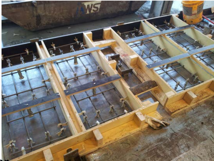
Rebar placement within molds
