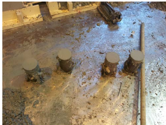
Rebar reinforcements in molds
